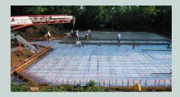
Benefits of post-tensioned concrete tennis courts include: Increased resistance to crack development, slab settling, and slab heaving; controlled slope for better drainage; demonstrated longer service life and lower maintenance costs; and minimization or elimination of control joints. Due to these benefits, post-tensioned concrete tennis courts provide the most uniform playing surface available.
